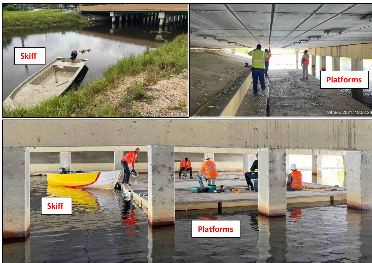
Figure 5 – Picture of “Work Skiff” and “Lightweight Canal Work Platform[s] – 5 FT x 8 FT”
